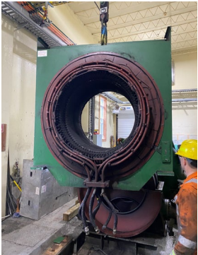
Lookout Brook generator stator being removed.
