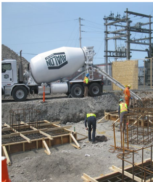
Foundations being poured for Islington Substation refurbishment.
